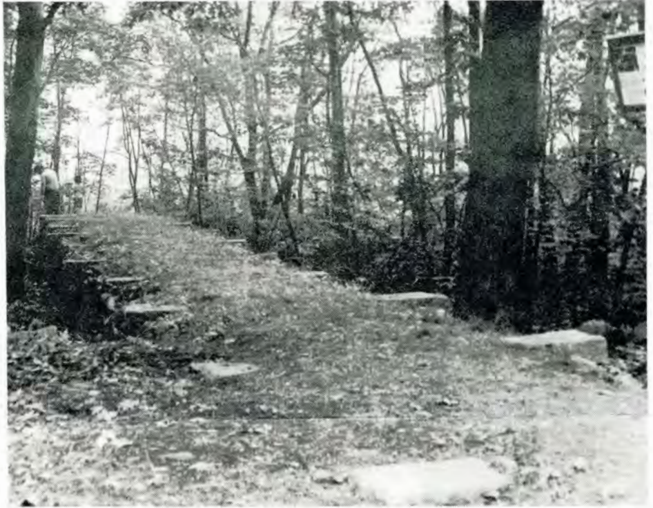
Bunker Hill Quarry end of the Granite Railway. This excavated 125 feet is complete except for the wooden rails. This portion of the railway was abandoned before wooden rails were replaced by granite.
